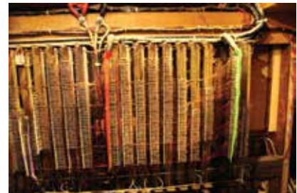
Filthy and very out-dated low-voltage wiring in the back of the console, laid out haphazardly. This is referred to in James Richardson-Jones' letter on 5th March 2009.
