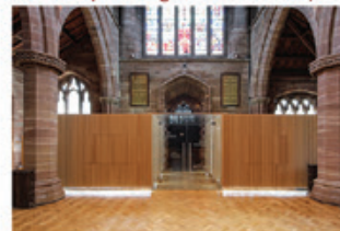
Acoustic panelling in South Transept
